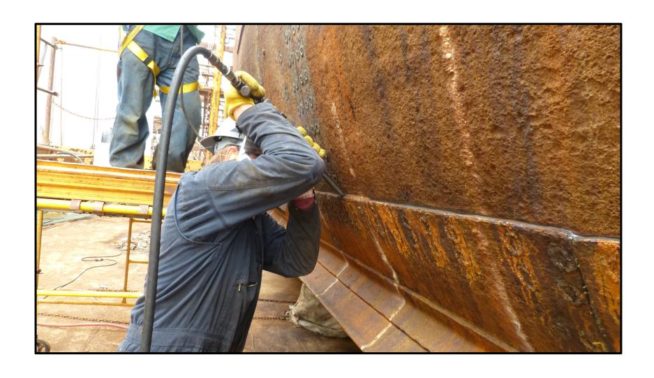
After drenching or re-riveting the plate, it is then "caulked" using a chisel point to peel over a sliver of metal to form a watertight joint.
