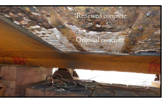
Rust stained concrete is material that was renewed during various repairs over the years.
