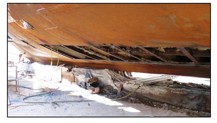
It is always difficult to gage what amount of cropping back will result in thick enough plate. When the plating in question is steel plate from the Greek restoration or Galveston first restoration, it is not a difficult decision. When it is the original historic wrought iron plate, the decision is more difficult, but in the end - it is whatever is best for the safe operation of the ship and her company
