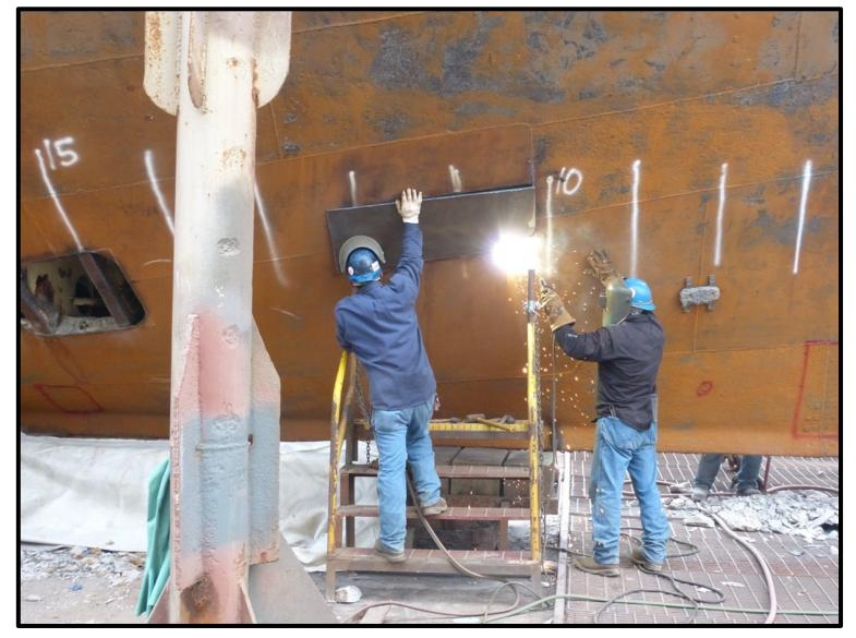
Fitting new plate insert section. Most of the hull plate renewals involved entire or large sections of A & B strakes and not smaller insert plates like the one above.
