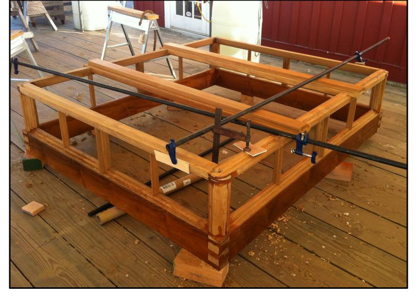
The new skylight being glued up and awaiting the new glass panels with an exact replication of original etched design.
