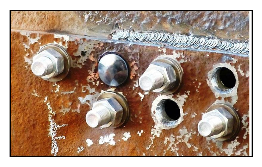
A shinny new rivet~ the rivet gun polishes the rivet point as it works the rivet in the chamfered hole. This is an example of a welded to rivet transition.
