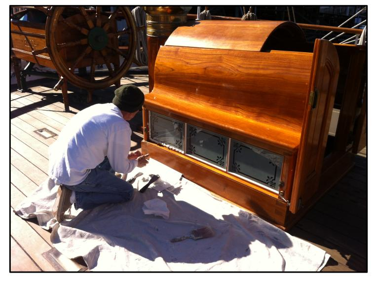
Glazing the new etched glass panels in the renewed aft companionway scuttle. We used Burma teak from the 1980 restoration of ELISSA to rebuild the skylight and scuttle.
