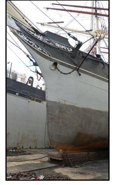
Sandblasting the hull before applying ceramic coating and bottom paint.
