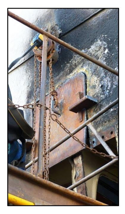
New steel plate in place and "dogged" - ready to be welded up before riveting new plate in space below.
