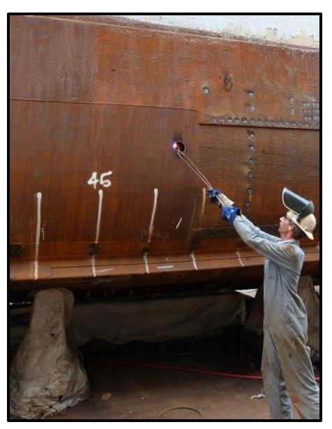
"Hot Rivet" is the cry as it is passed through a hole cut into the hull. This hole will be welded closed later.
