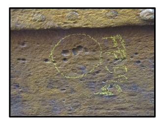
Electrolytic corrosion resulting from Hurricane Ike
