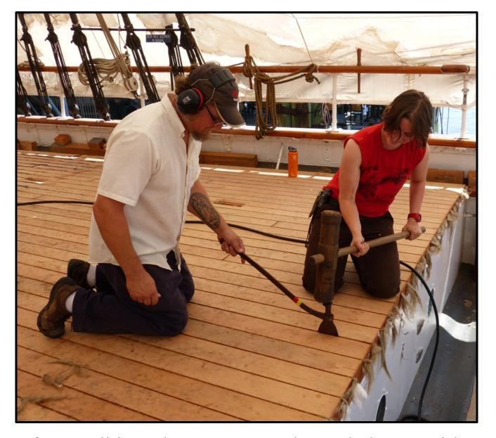
After caulking, the seams are "horsed" home with a large mallet called a Beetle.
