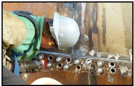
Plate bolted up ~ rivets are placed in empty holes and then the bolts are removed and the remaining rivets passed.
