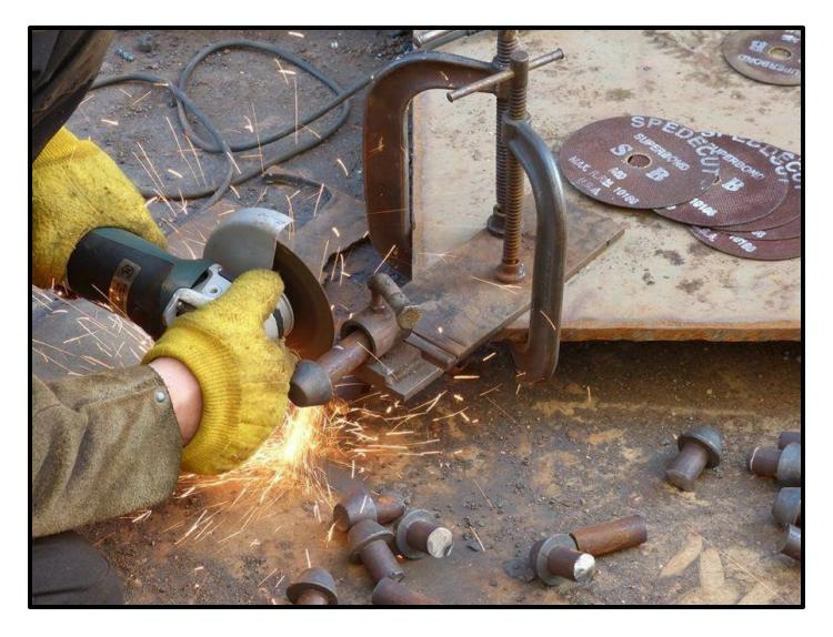
Cutting new rivets to proper length ~ each one is slightly different in length.
