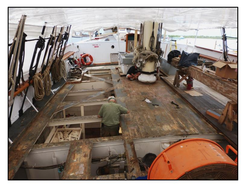
Dressing the steel plate on main deck, before painting steel and laying new decking.
