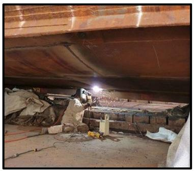
Shipfitters and welders needed to be limber to weld up plate in tight and cramped spaces
