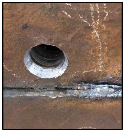
New rivet hole drilled and reamed in renewed steel plate before riveting.
