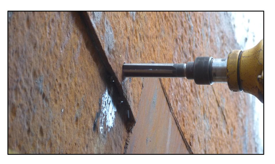
Reaming out old rivet hole for new rivet.
