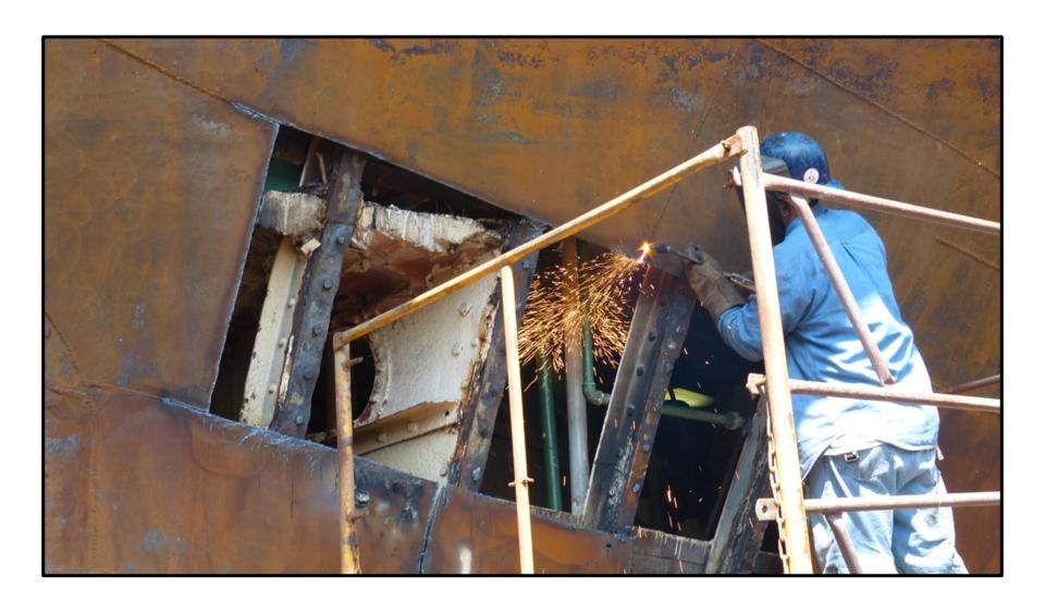
A good welder can wash off a plate and barely mark the frame underneath.
