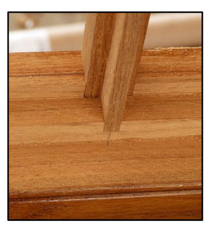
Hand-cut dovetails in 3" thick teak with exquisite detailing.
