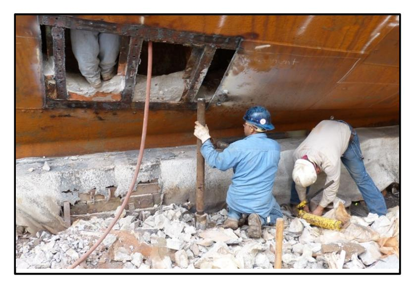
Breaking out concrete ~ over 22,000 lbs. was removed.
